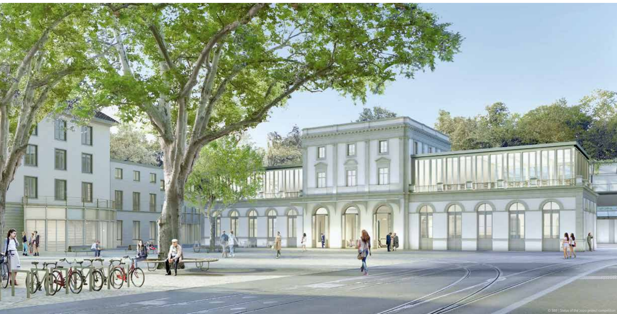
Passengers reach the completely remodeled station via the forecourt.
