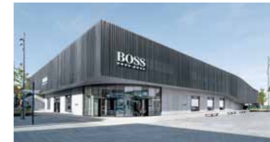
The new HUGO BOSS flagship building in Outletcity Metzingen sets a new standard in terms of design and sustainability.
